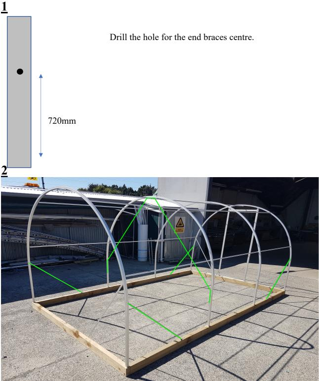
This picture shows the locations for the 4 end braces and a suggested position for the braced arch. The braced arch should be positioned as central as possible within the tunnelhouse.
