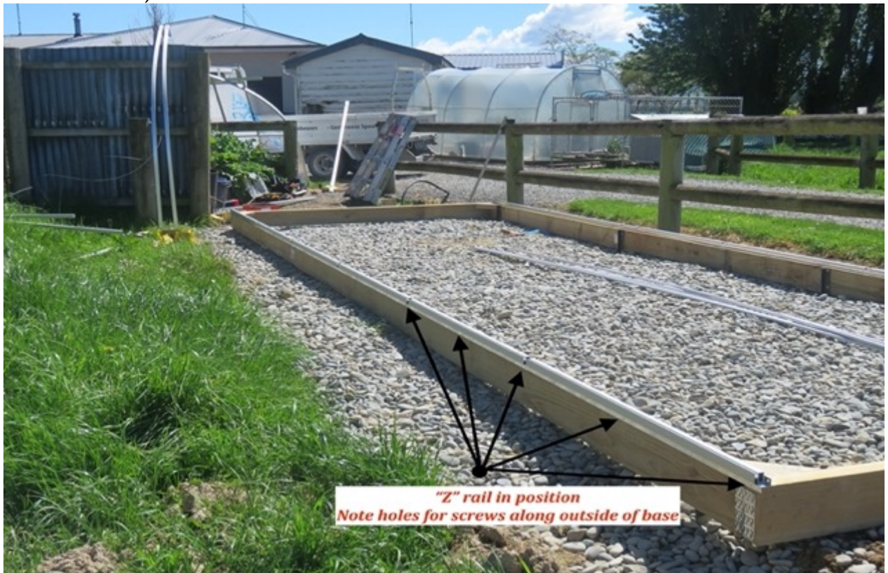
B) TIMBER BASE WITH 'Z' RAIL IN POSITION
