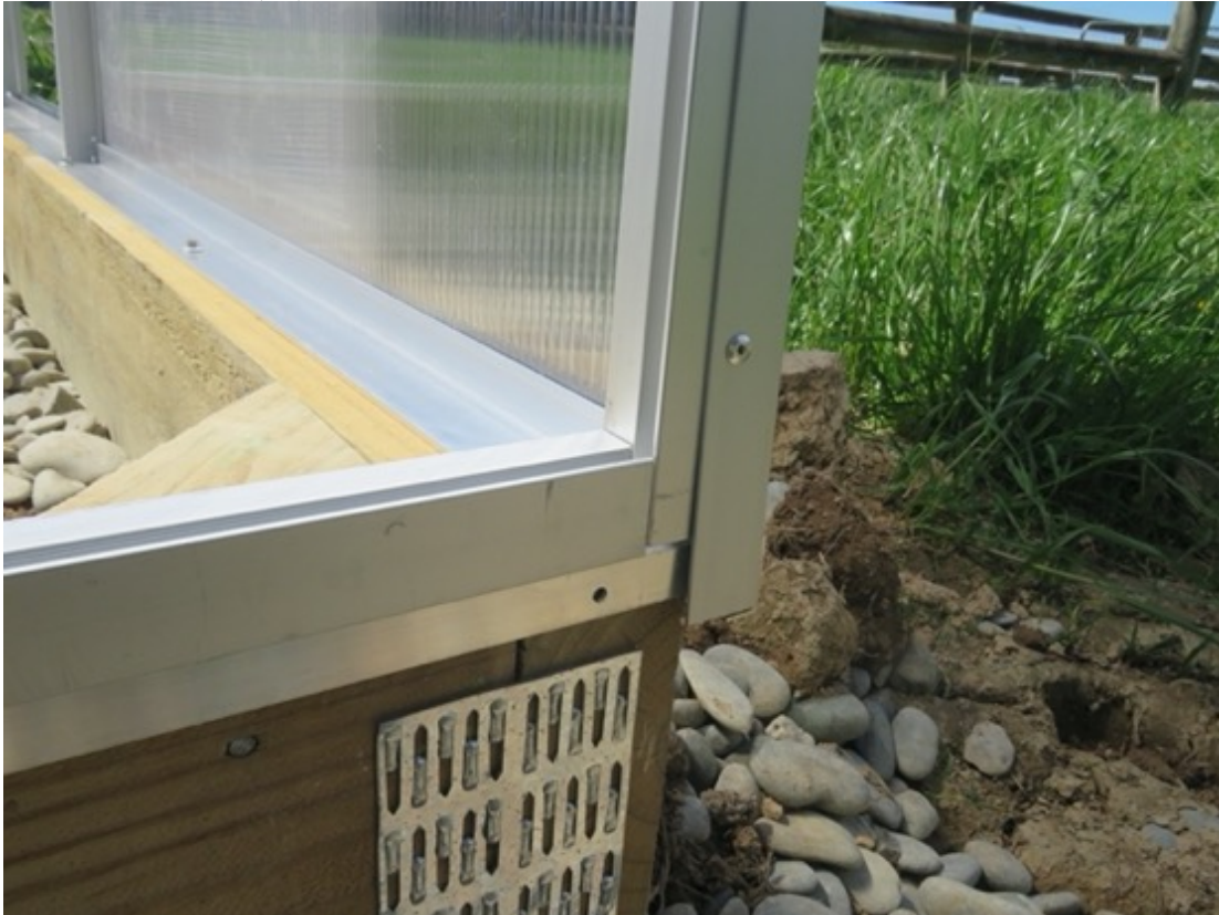
(C) END-WALL SLOTTED TO 'Z' RAILS
