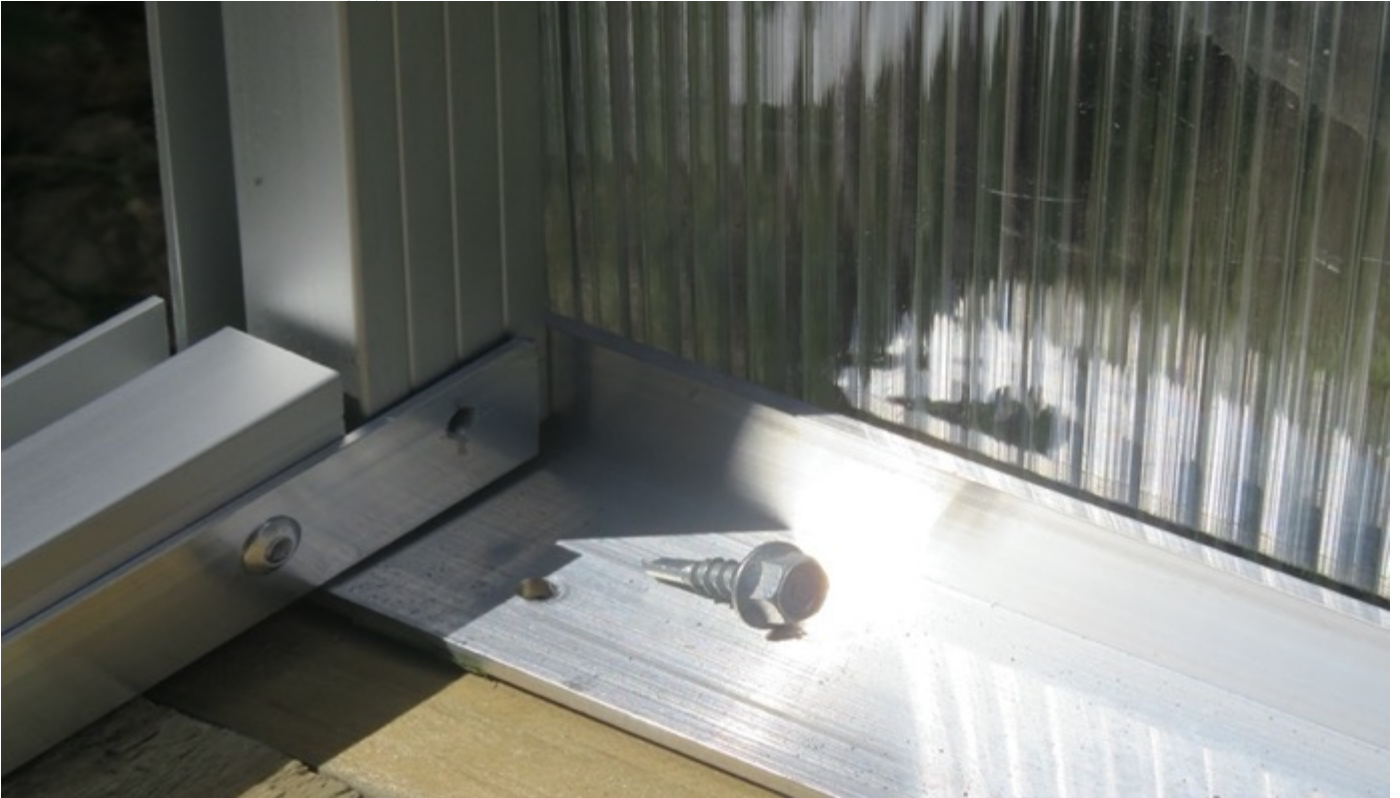
(F) ATTACHING END-WALLS TO 'Z' RAIL
