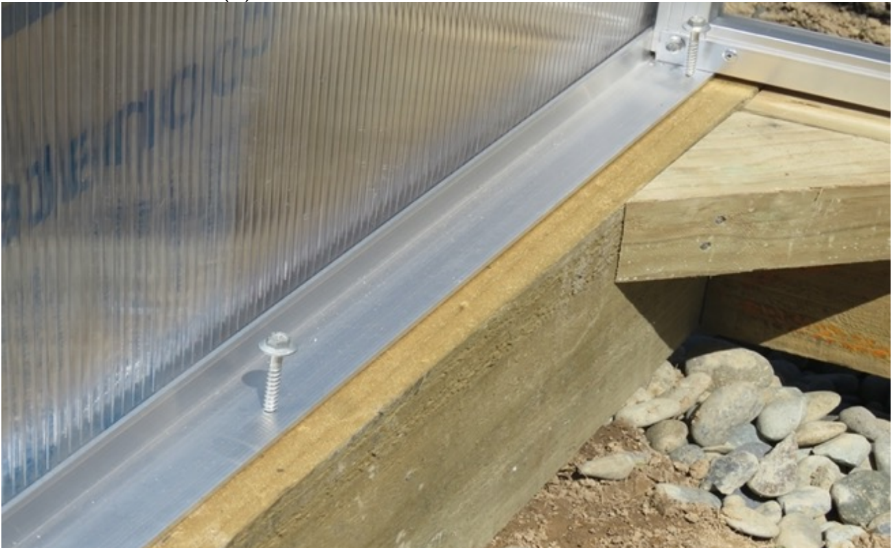
(F) ATTACHING END-WALLS TO BASE
