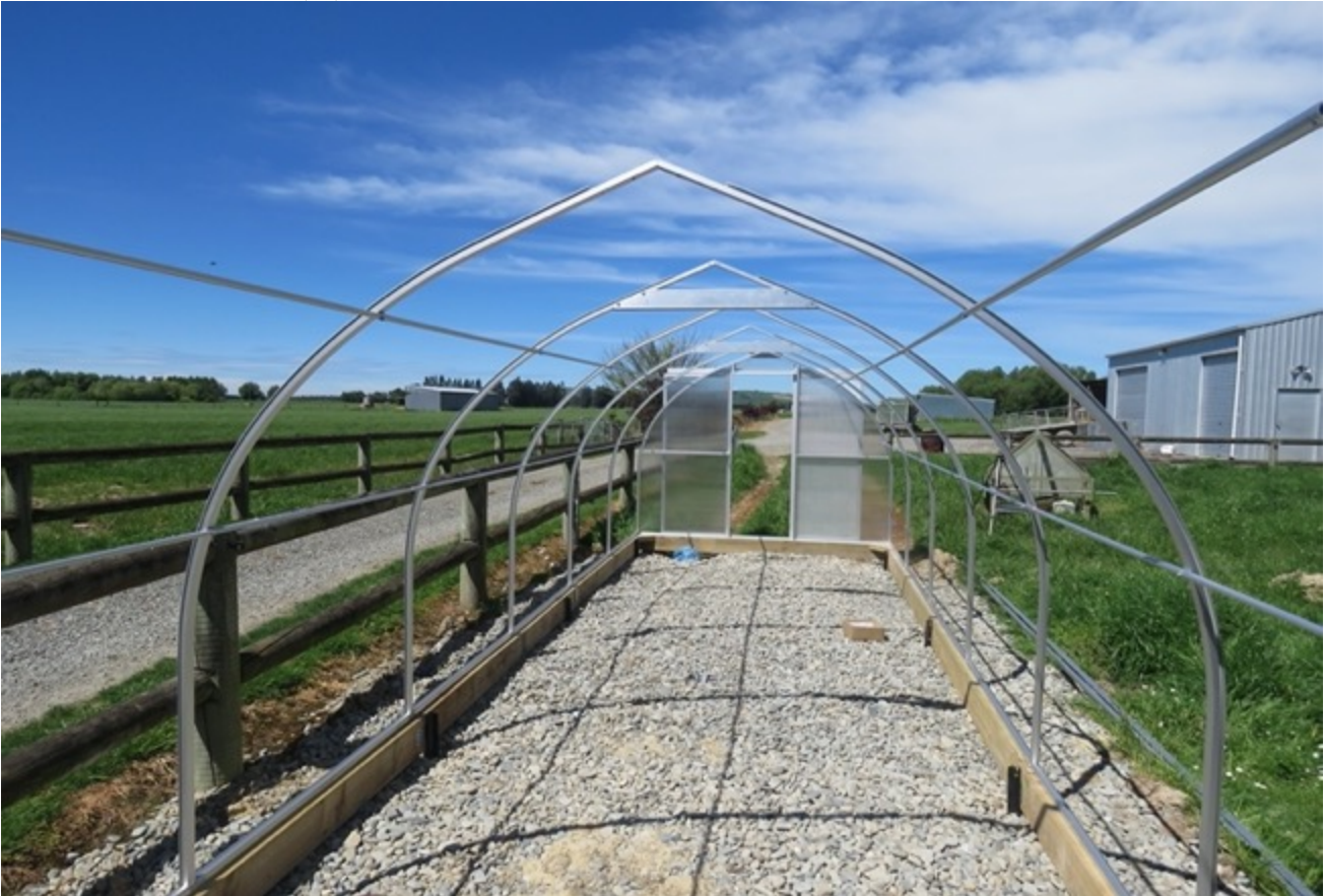
(E) ATTACHING PURLINS TO END-WALLS
