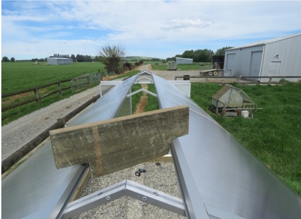
(J) USING SPREADER BAR
