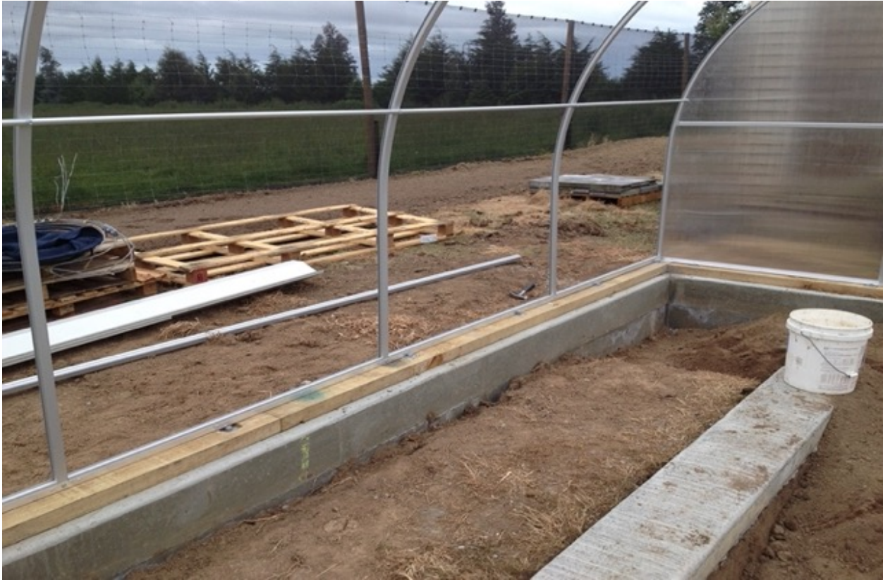
A) CONCRETE NIB WITH TIMBER TOP
